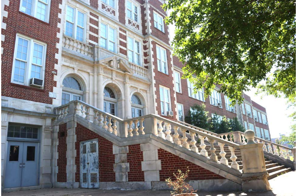
North entrance- Detail 3
