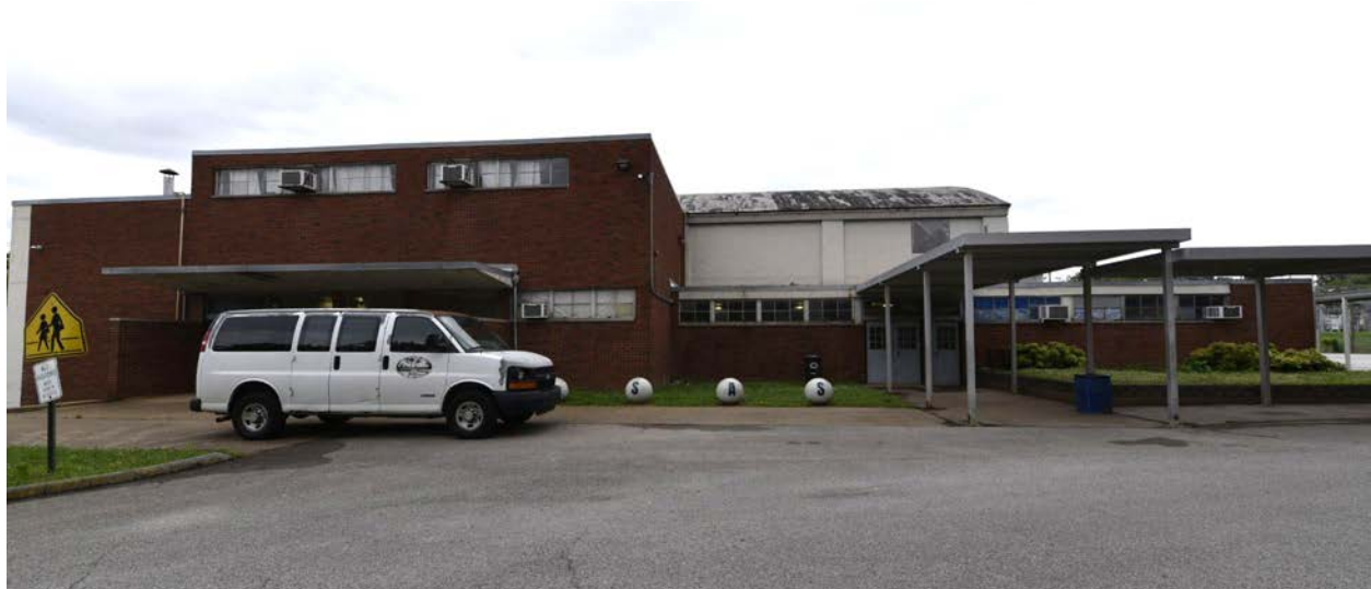
North elevation- Gymnasium
