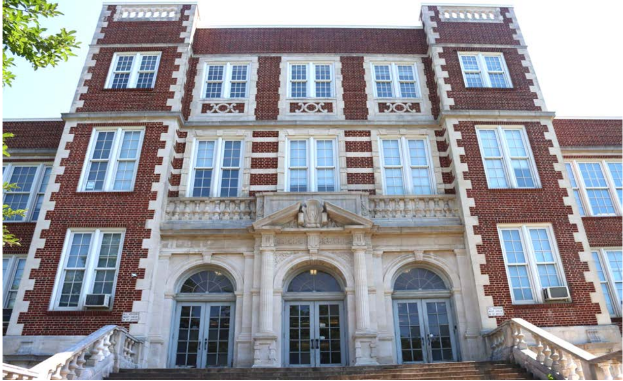
North entrance- Detail 1
