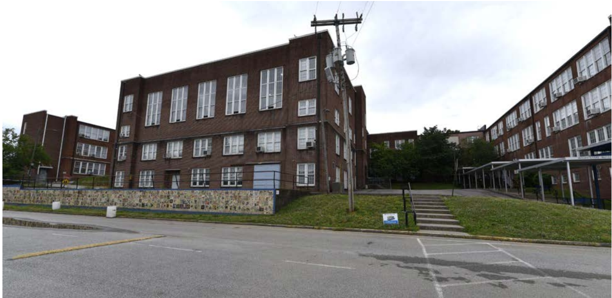
South oblique- Wing B (center) and Wing C (right)
