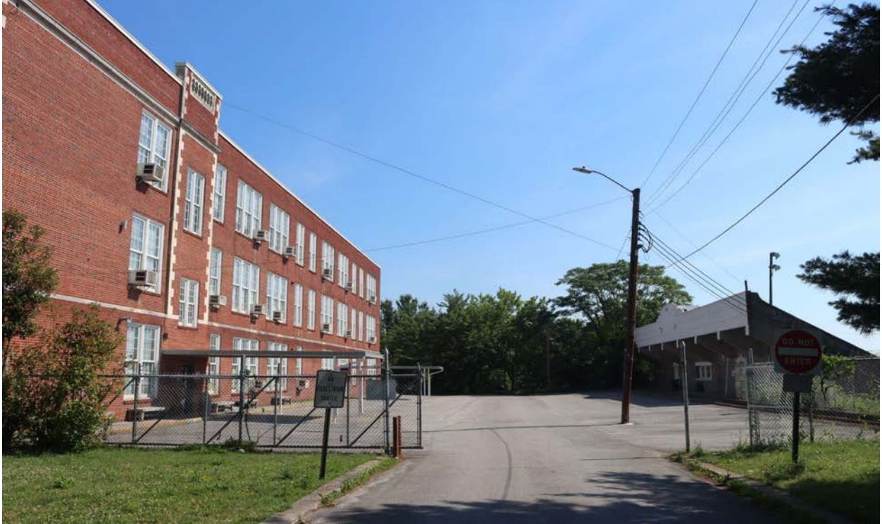
West oblique- Facing stadium and field
