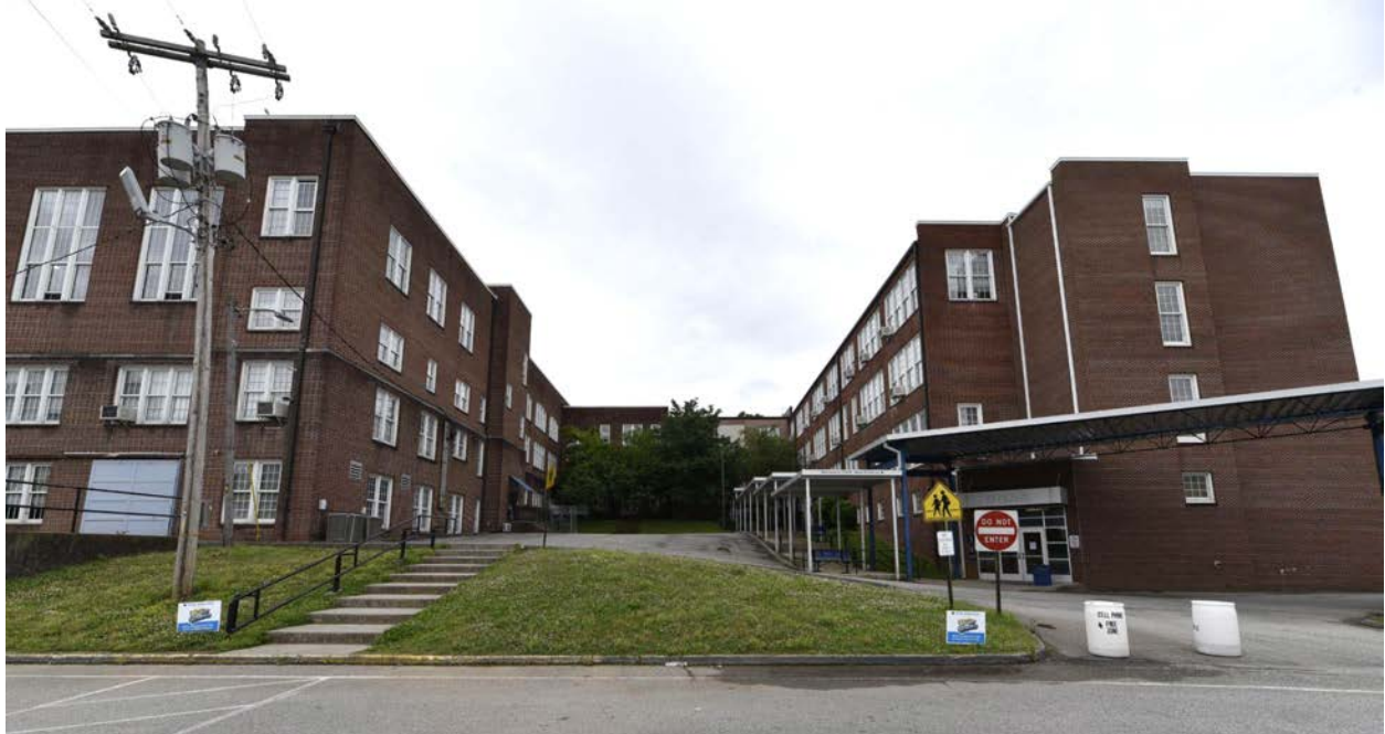
South elevation 2- Wing B (left) and Wing C (right)
