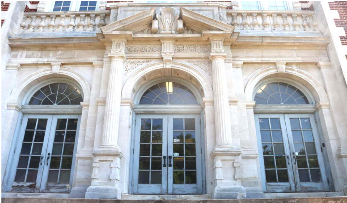
North entrance- Detail 2
