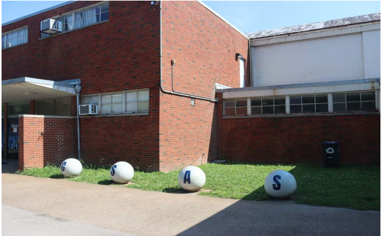
North details- Gymnasium entrance
