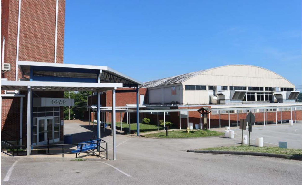
Awning detail - Connecting Wing C to John B. Steele Gymnasium
