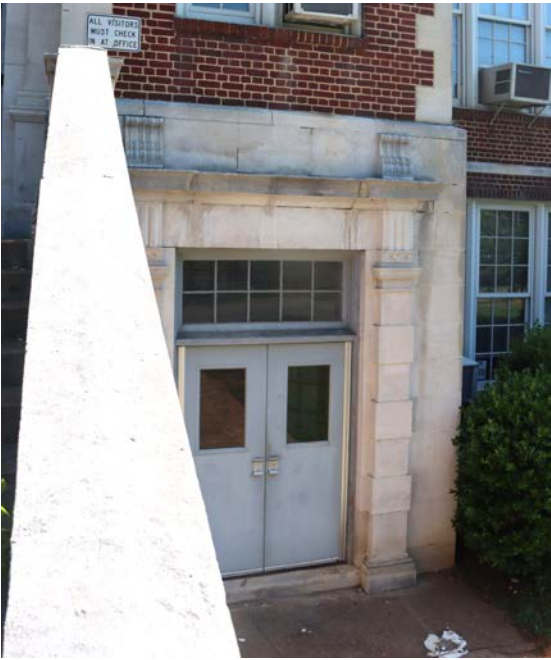
North entrance- Detail 4
